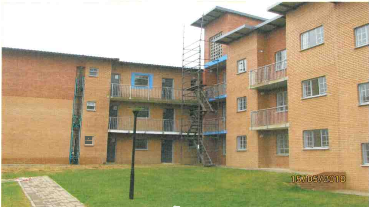
Figure 1: Photo: Turffontein Social Project in the Inner City
